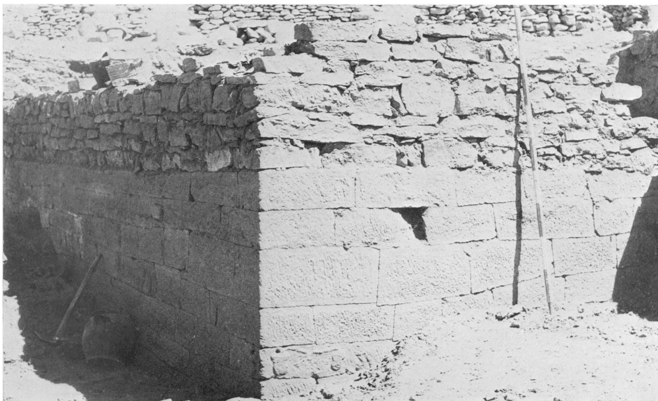
2. North-west corner of the Meroitic building
