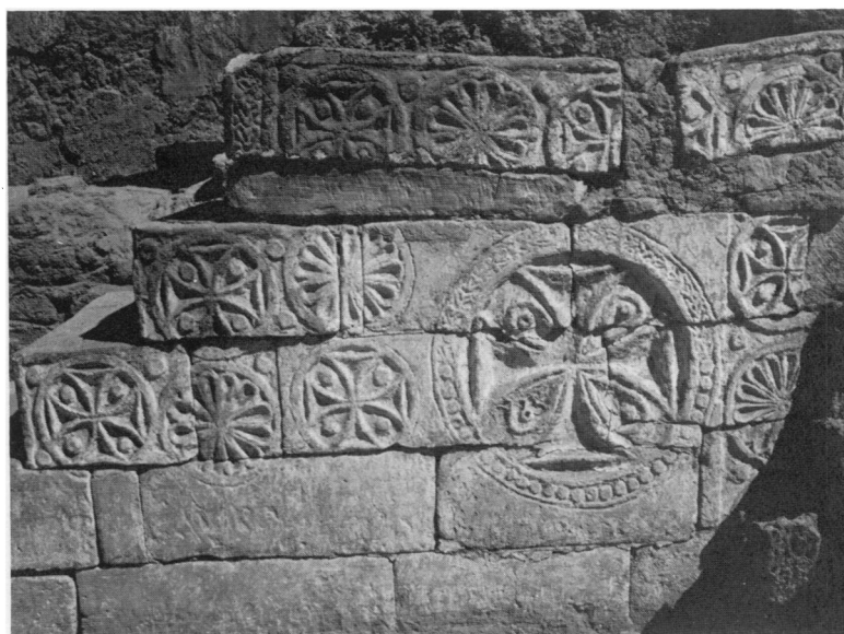
4. Ambo . Stump of wooden pillar of triumphal(?) arch in right foreground
