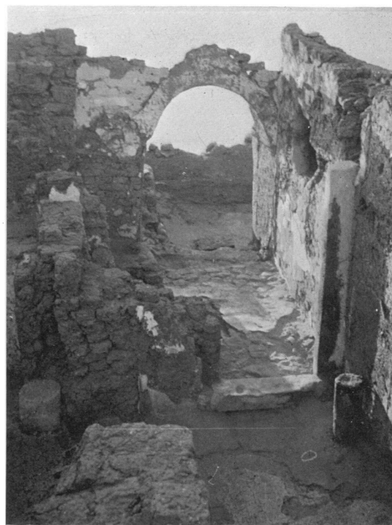
3. Entrance to baptistry from south aisle (B). Room L to rear, looking east
