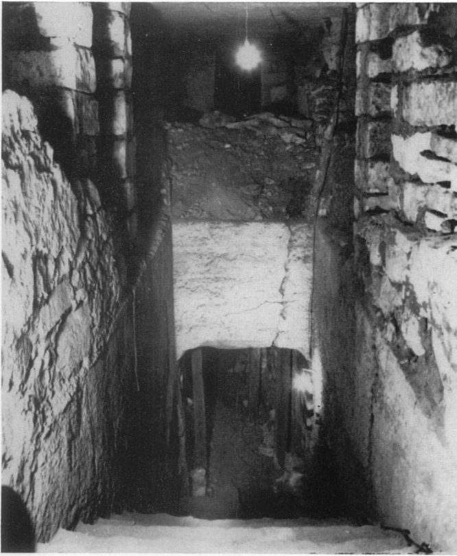
1. Stairway connecting the upper and lower galleries, from above
